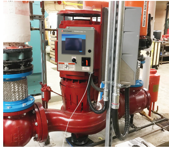
Series e-80SC pump installed with Technologic variable speed drive and Technologic PPS controller
